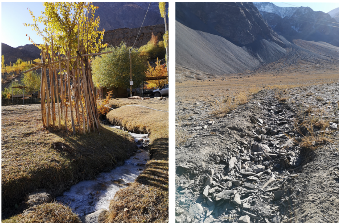
Figure 35: Functioning and destroyed irrigation channels in and around Barchidev village
